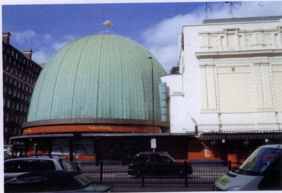
Marylebone Road – View of Existing Elevation
